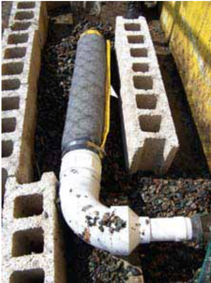
Pad mount install.
