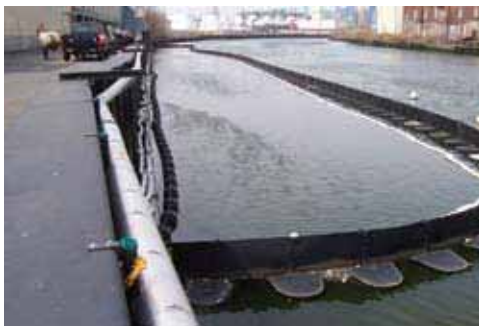
Polypropylene Boom to be replaced at Newtown Creek.
